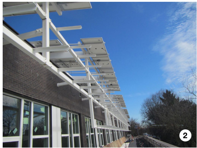
Photo 1: View southwest in the Grand Open Common Space inside Building F. Progress continues with the glass curtain wall in place, Sheetrock and duct work are ongoing. Photo 2: Solar panels installed above the outdoor observation deck on the south side of Building H and overlooking Buckman Field. (Photos courtesy of Gerry Ochs.)
