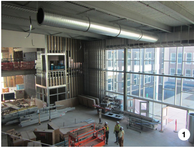
Photo 1: View southwest in the Grand Open Common Space inside Building F. Progress continues with the glass curtain wall in place, Sheetrock and duct work are ongoing. Photo 2: Solar panels installed above the outdoor observation deck on the south side of Building H and overlooking Buckman Field. (Photos courtesy of Gerry Ochs.)
