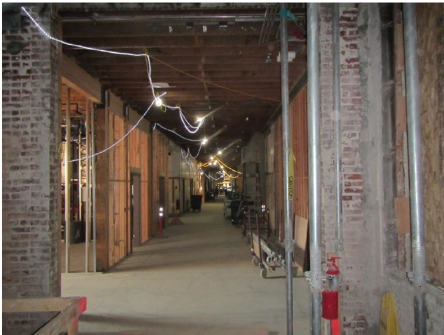
Left photo, top: View SW as construction crew works on seismic upgrades for the new roof system over the Old Gym. The upgrades are similar in scope to the roof replacement on the school's main building, Building E. Left photo, bottom: View from outside the auditorium, looking south down the hallway of Building E at ground level. The concrete floor is now in place and wall framing is in progress. Right photo, top: Progress on assembly of steel framing components for Building H. The view is SW and Buckman Field is off to the left. Right photo, second: The construction tent has been removed and the new roof is complete on the Building E. Right photo, third: View east from back side of the auditorium showing progress on Building B, located along Irving Street between the auditorium and new Building C. The lower level of Building B will house the New Band Room. Right photo, bottom: All new electrical, duct work and fire protection systems are underway in Building E.
