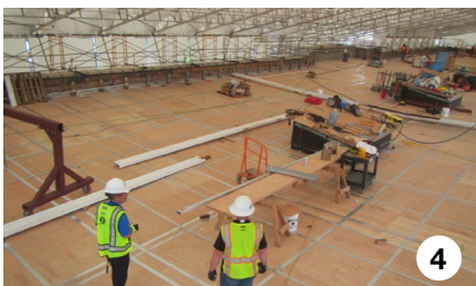
Photo 1: New community room for variety of gatherings at Benson Tech. Photo 2: The Learning Stairs in Building F Grand Common Space, temporarily supporting scaffolding for installation of overhead work. Photo 3: Re-purposed old growth timber beams were converted into benches for placement in the school corridors. Photo 4: Mass plywood sheets installed on the roof with hurricane straps and metal beam framework for seismic restraint. Photo 5: Main piping for the hydronic piping system is stubbed up inside Building H for connection to the future hydronic heat transfer unit. Photo 6: Solar panels installed above the outdoor observation deck on the south side of Building H. (Photos courtesy of Gerry Ochs)
