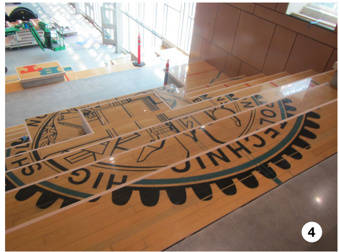
Photo 3: The completed restoration of the Old Gym with new court floor and upper running track. The gym is now designated as G1. Photo 4: Existing gymnasium flooring with Benson Tech gear logo re-purposed to create the seating surfaces for the Learning Stairs located in the Building F common space. (Photos courtesy of Gerry Ochs.)
