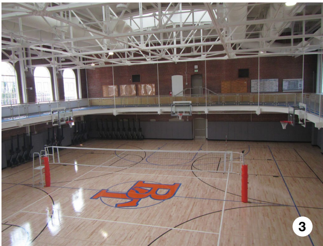
Photo 3: The completed restoration of the Old Gym with new court floor and upper running track. The gym is now designated as G1. Photo 4: Existing gymnasium flooring with Benson Tech gear logo re-purposed to create the seating surfaces for the Learning Stairs located in the Building F common space. (Photos courtesy of Gerry Ochs.)
