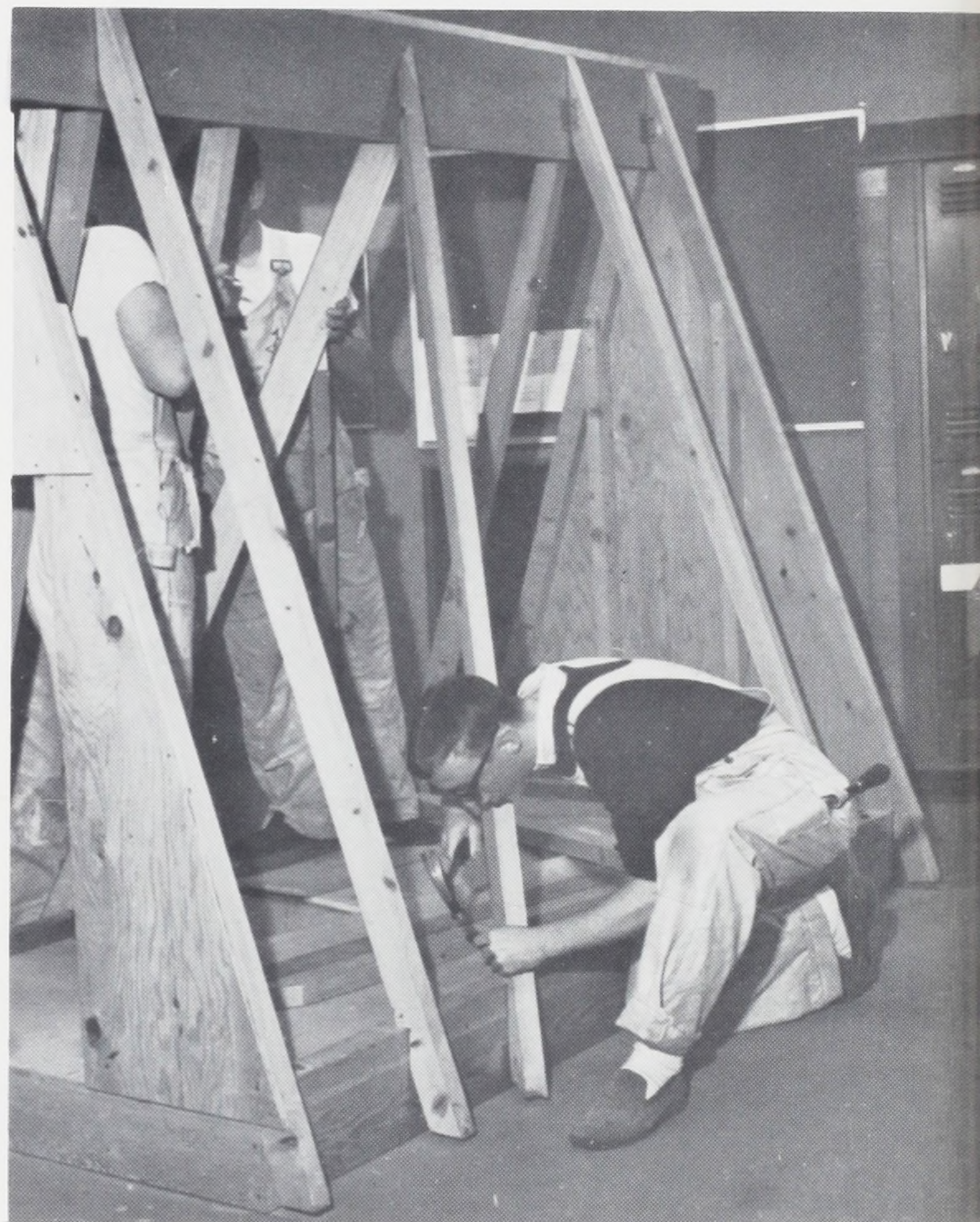
John Brill, above, nails down a valley rafter on a miniature double-A-frame house. Ron Sherman and Carl Nolten stand busily at work in the background.
