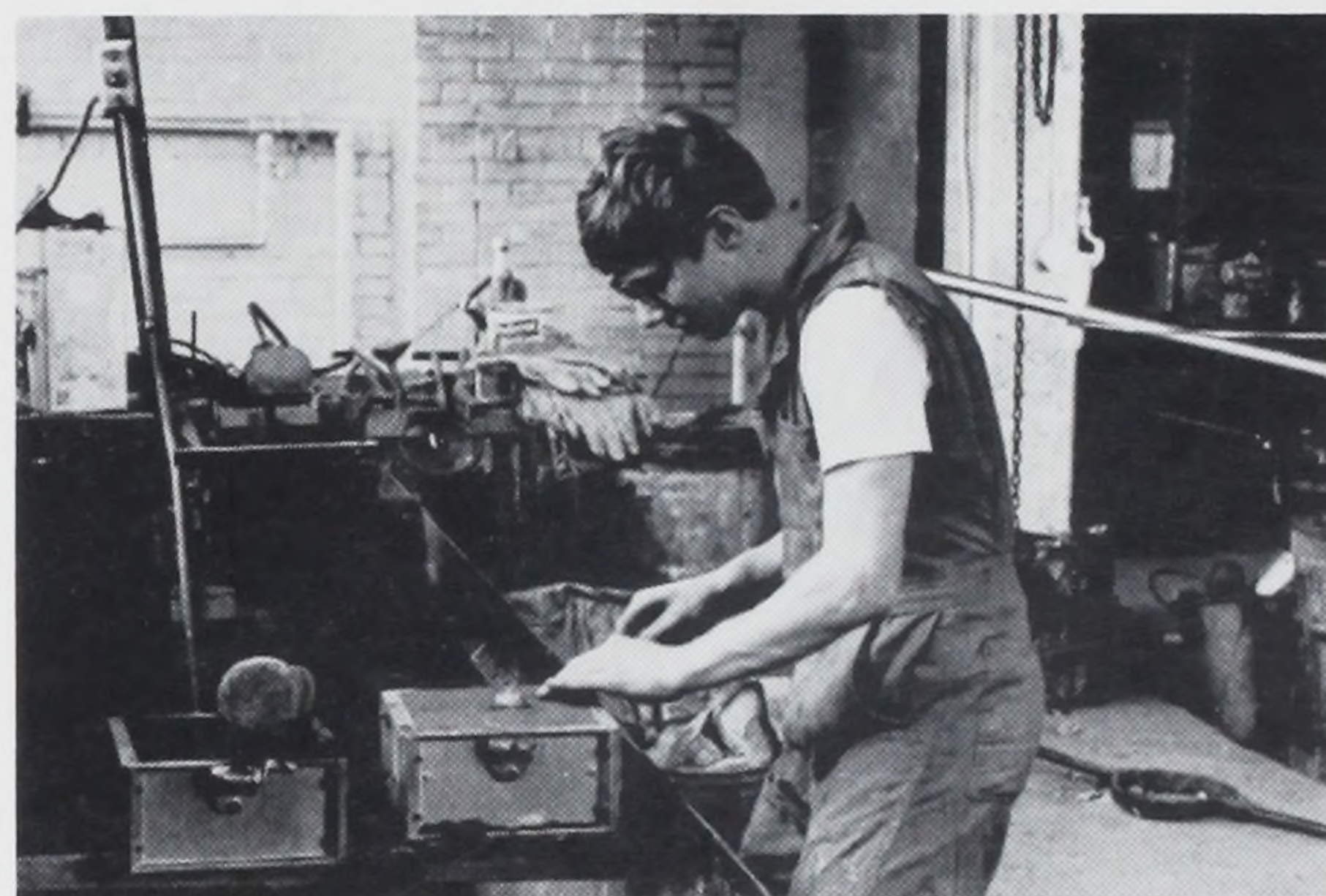
Bill Schouten, a Benson Foundry major, is smoothing a mold.
