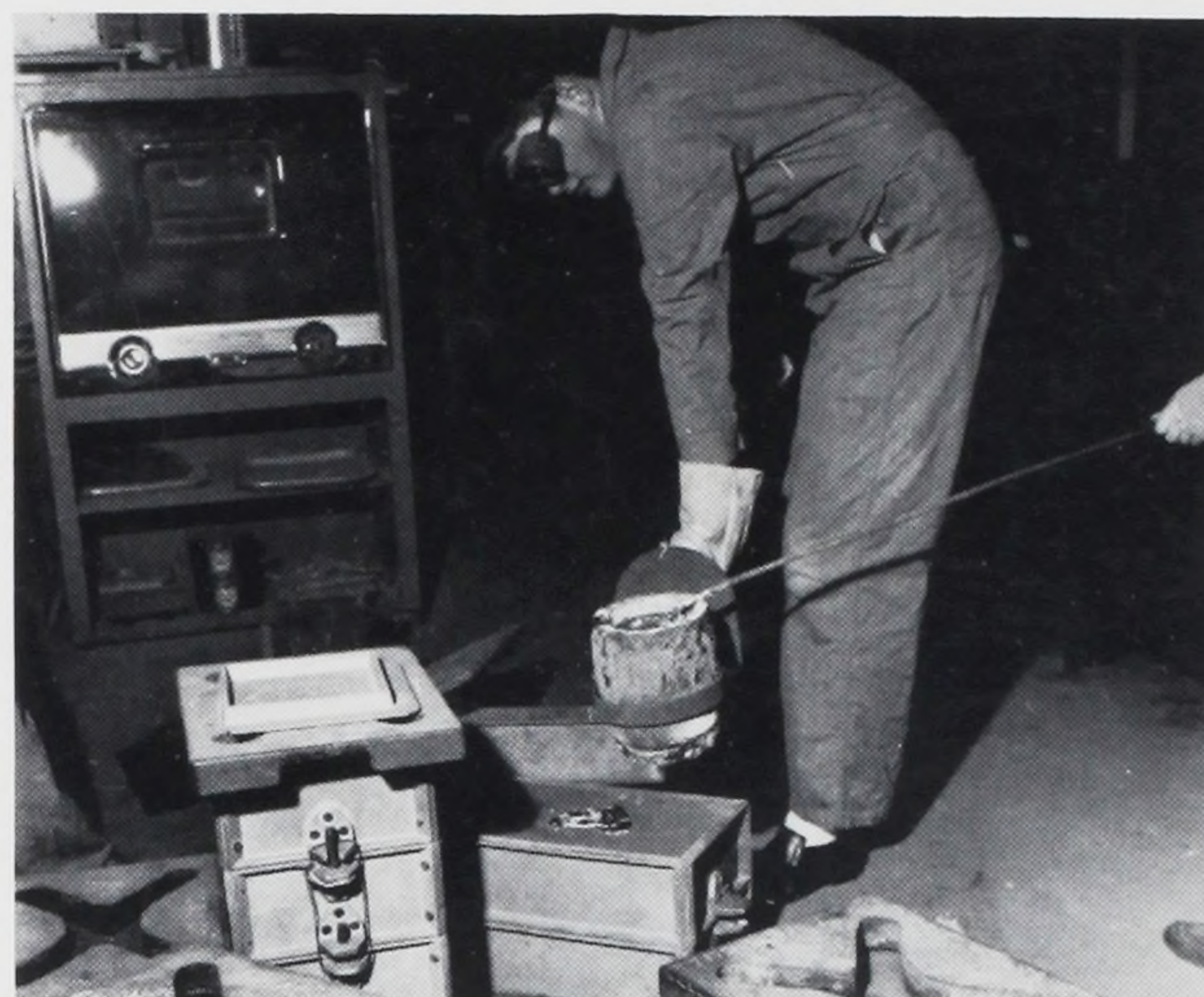
Student in Foundry gets helping hand from buddy while pouring molten lead into mold; small kiln is in background.
