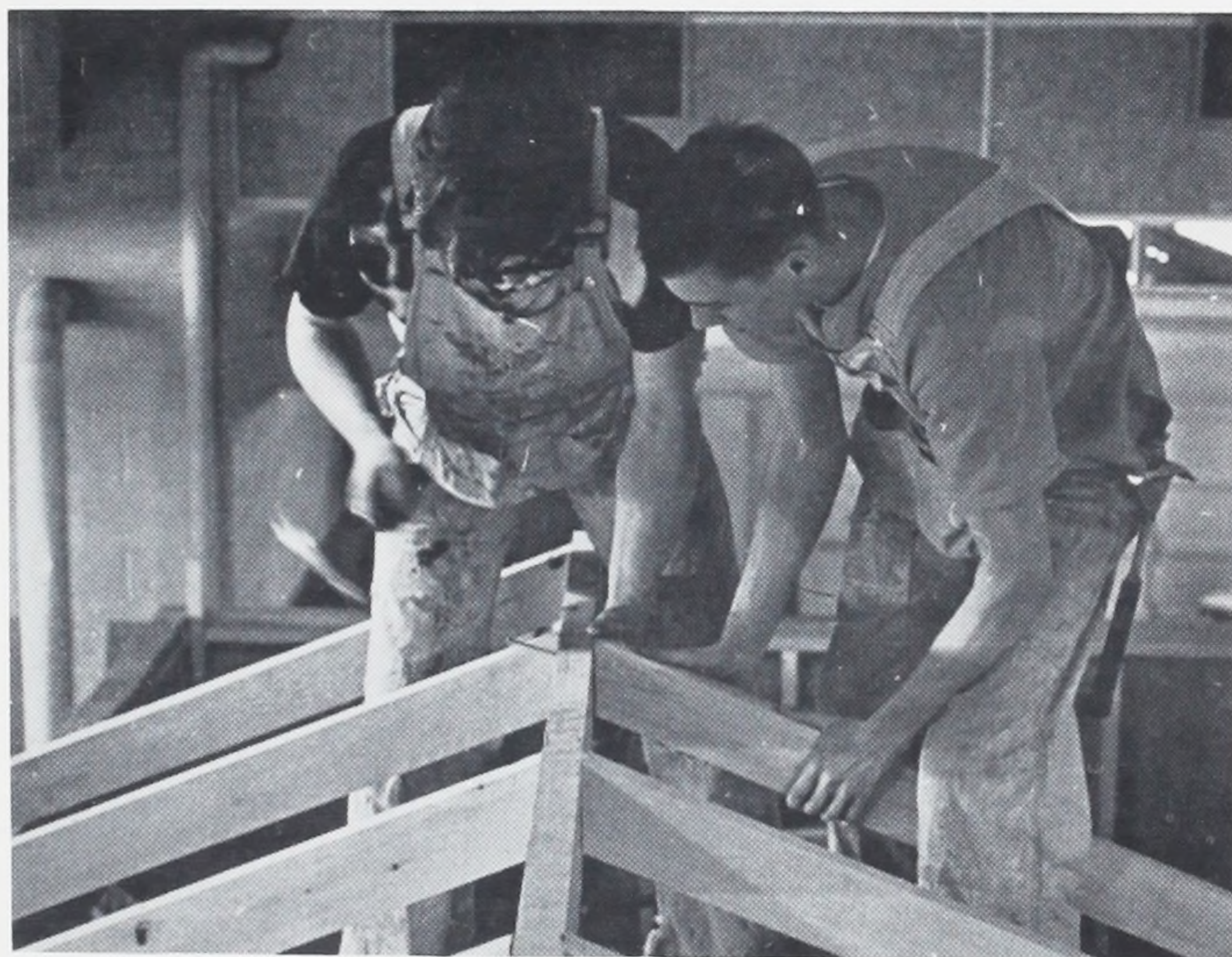
Walt Bahr and Richard Reitz install Rafters on house which is built each year in Building Construction.
