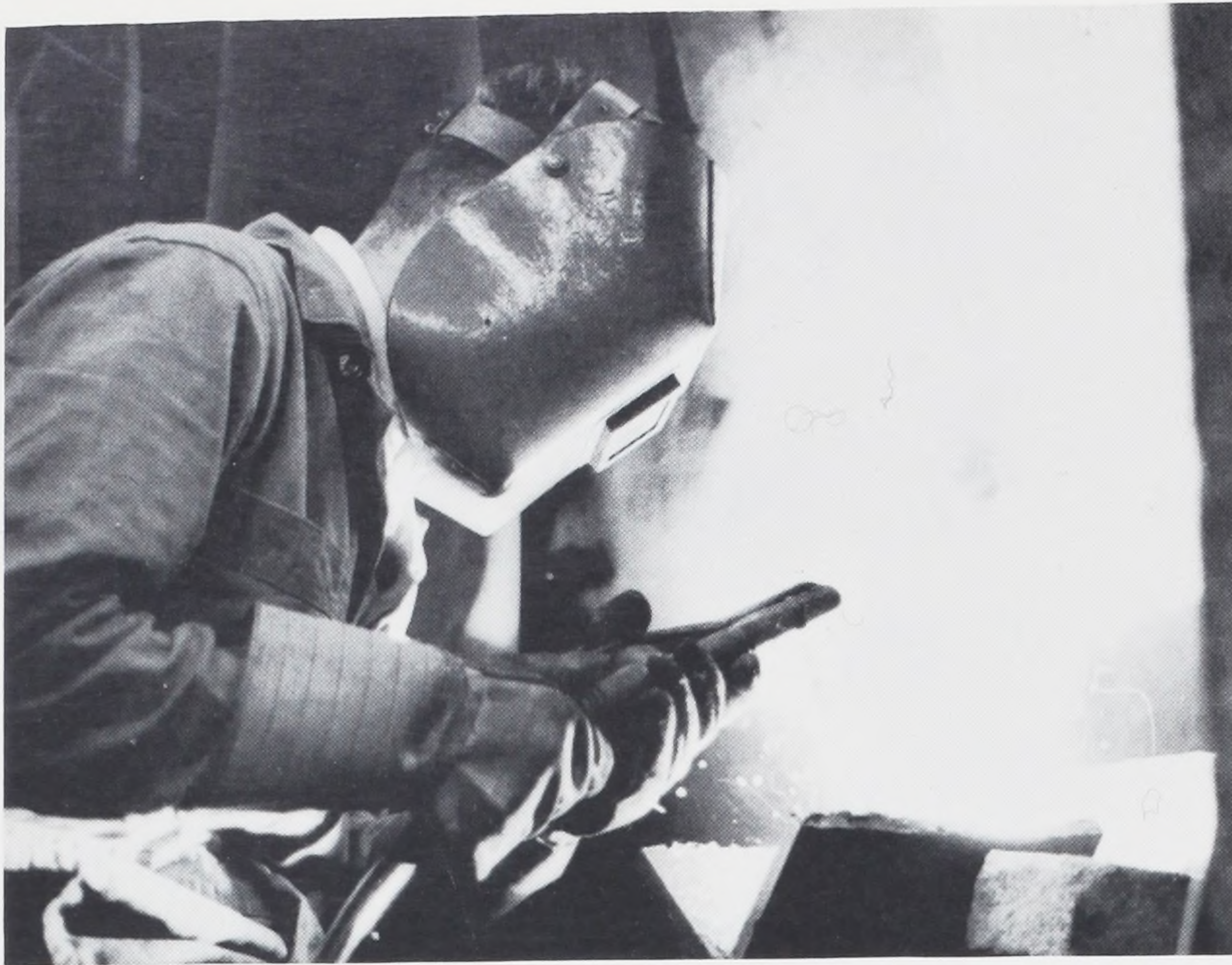
Student in Welding shop working on a flat fillet weld.
