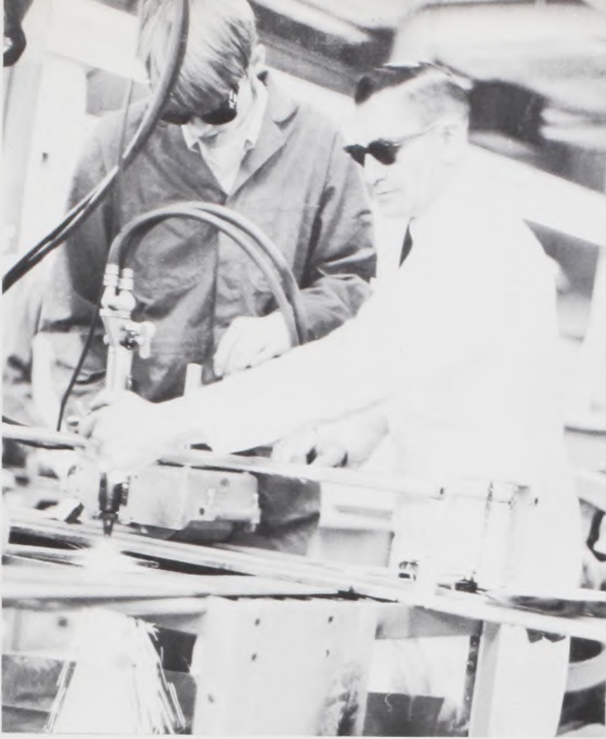
Instructor Mr. John Milovich instructs student Keith Harrington on use of the automatic cutter.
