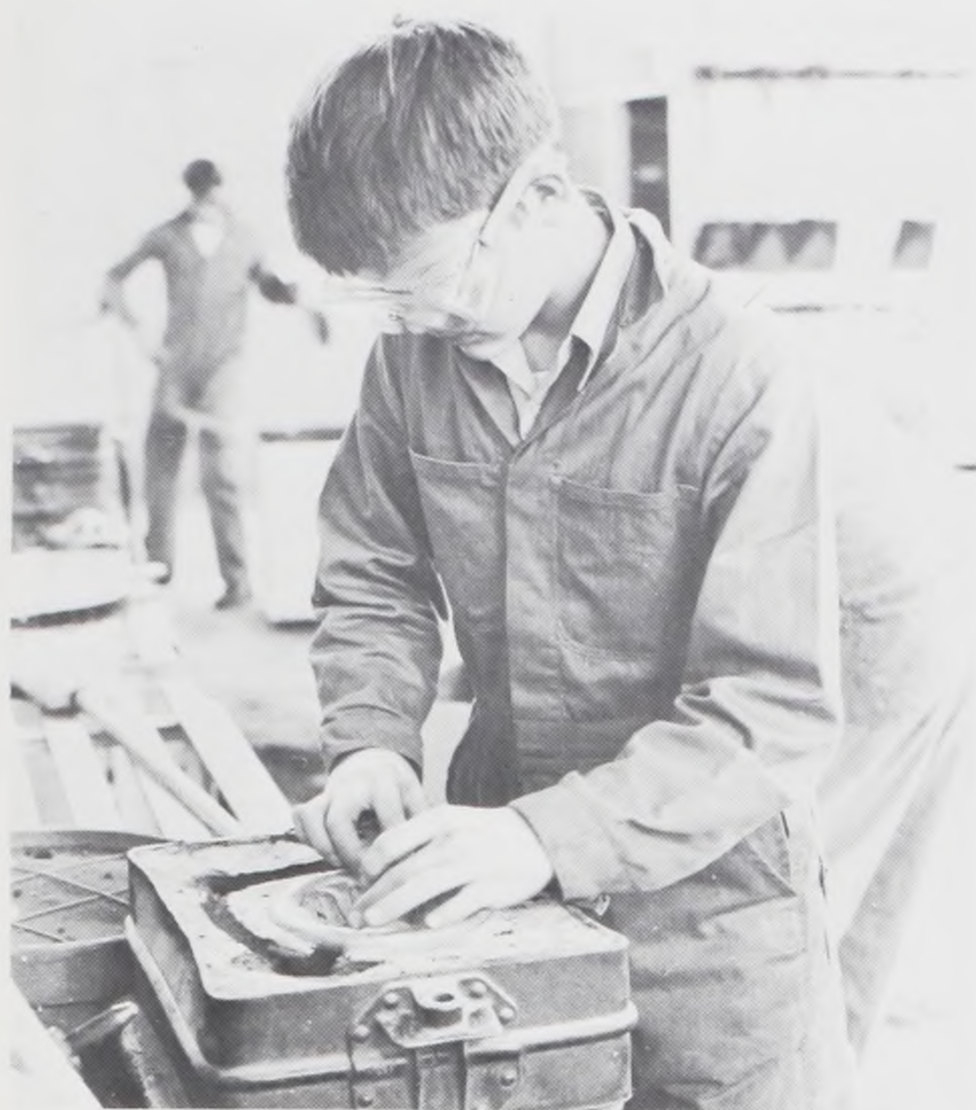
Student removes a pattern from the sand mold.
