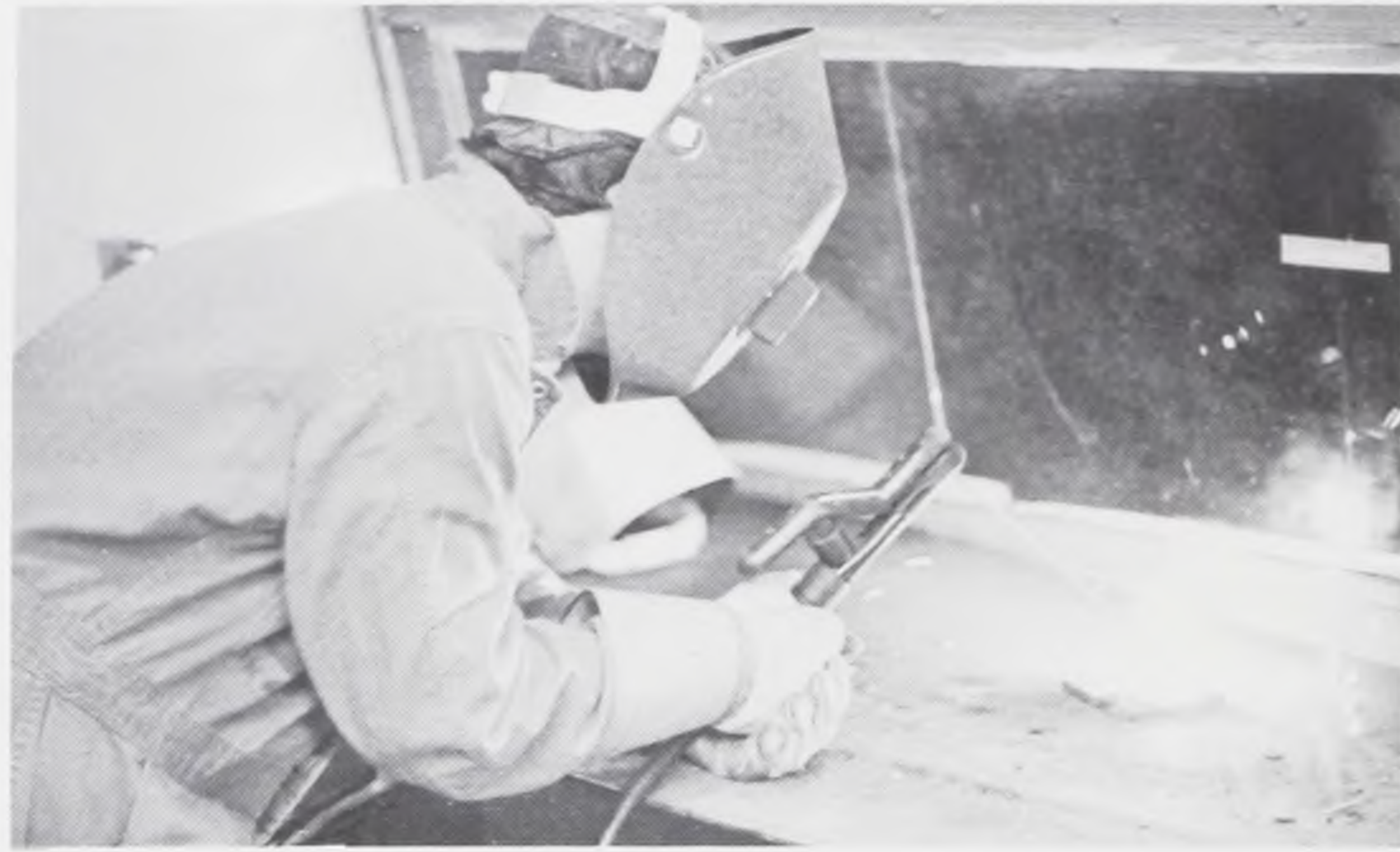
A sophomore student runs a few "beads" with an arc welder.
