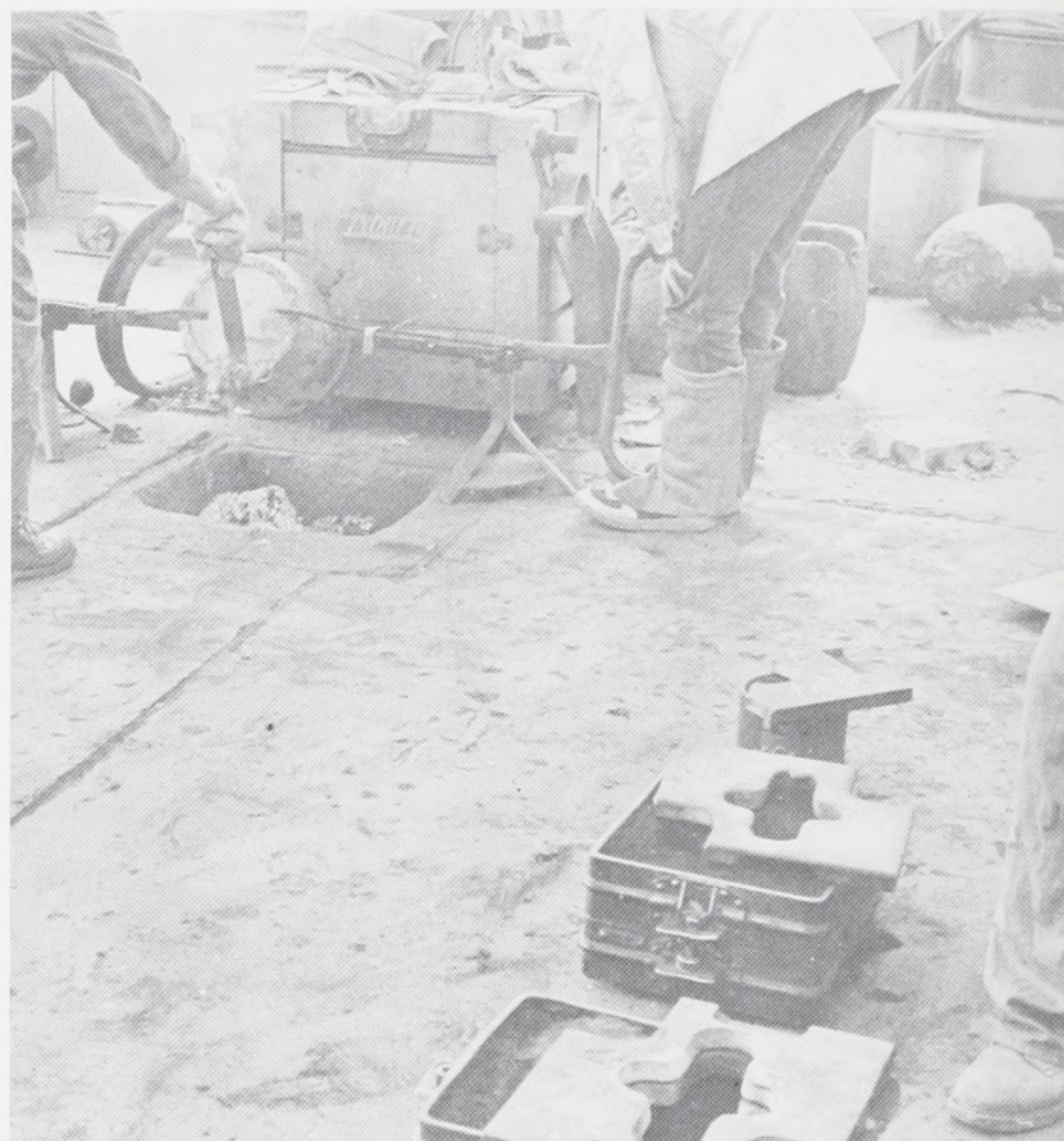
A. Julianne Trout (10) sands on wooden pattern form for her class project. B. After metal is poured the remaining metal must be emptied. C. Brass bells, trophy plaques, clock bases were among the many projects on display on two long tables during the Tech Show.
