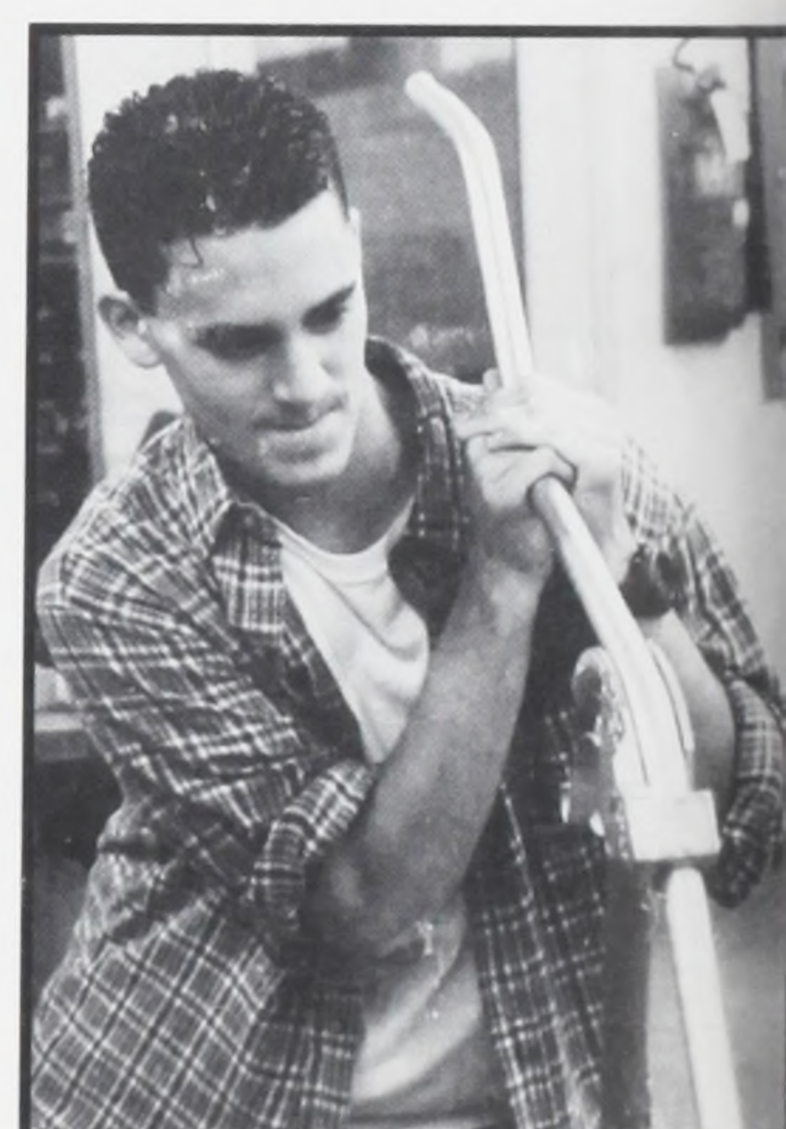
Nick Trujillo bends conduit into saddle.
