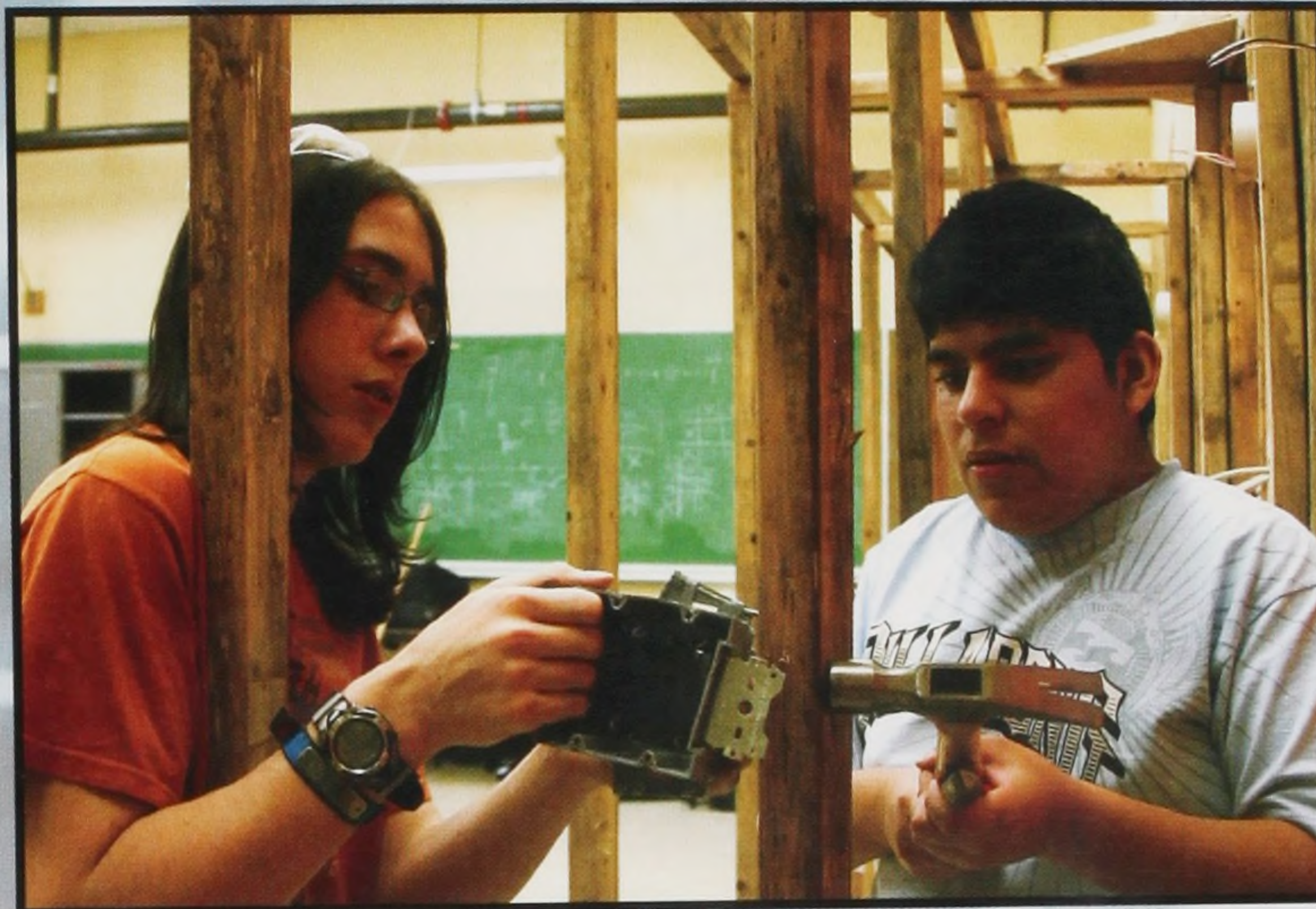
Ethan Dedrickson and Drake Drawley install a switch box into a wood plank. They have to be careful not to break the plank or the whole frame will be unusable.
