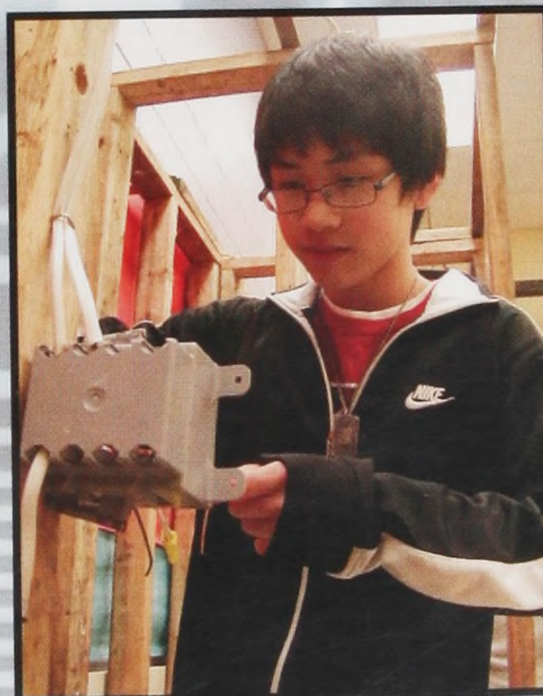
Duy Nguyen finishes his wiring project in Sophomore Electric. He has to insert the wires into the boxes, while making sure all the wires are connected and in the right locations.
