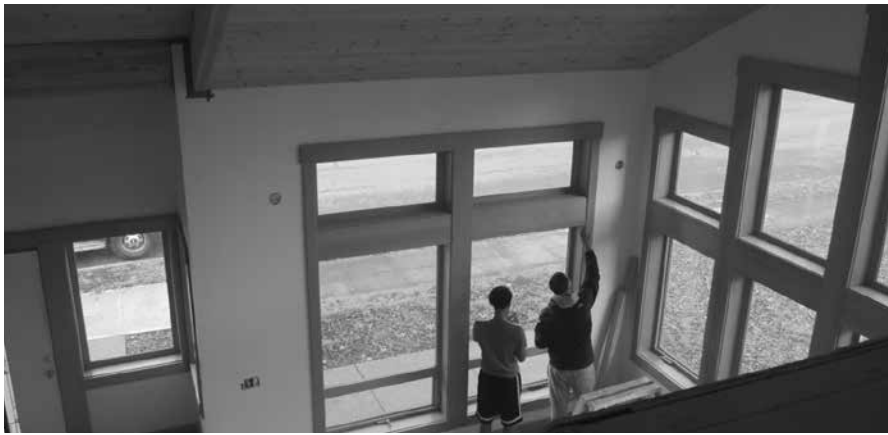
Benson Tech students at work in the 2014-2015 house construction.
