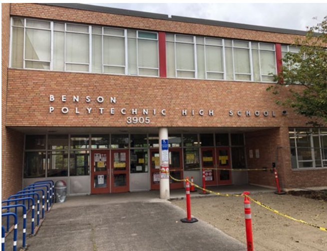
Above: New signage on the entrance of the former Marshall High School campus, which Benson Tech faculty and staff will call "home" for the next three years while the Benson Tech campus modernization project is under construction. Photo courtesy of Portland Public Schools/Curtis Wilson.
