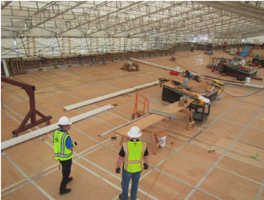
Photo at left: Mass plywood sheets installation on the roof with hurricane straps and metal beam framework for seismic restraint in progress. Top photo right: Progress on seismic upgrades of the old gym. Note the steel beams on the floor will be affixed on the inside face of the exterior brick walls. Bottom photo right: Main hallway looking north from just outside of the gym breezeway. Welded metal pan decking in place for casting a 6-inch-thick concrete floor.
