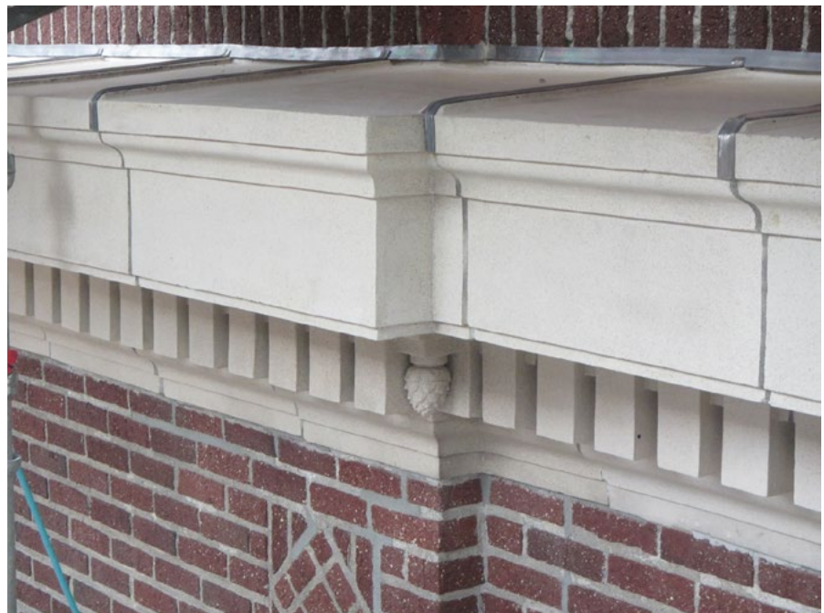
Photo at left: Example of an interior shear wall constructed using the shotcrete method. Top photo right: View from the roof looking east at progress on the foundations and slabs on grade for the new two-story Building "H." The radio station building is in the background and Buckman Field is on the right. Bottom photo right: The terra cotta trim and brickwork have been sandblasted using soda powder to restore the appearance. New jointing and flashing has been installed between the terra cotta sections. Note the detailed pine cone feature underneath the corner.
